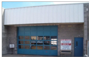
Exterior Garage Door – Before
