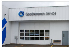
Exterior Garage Door – After
